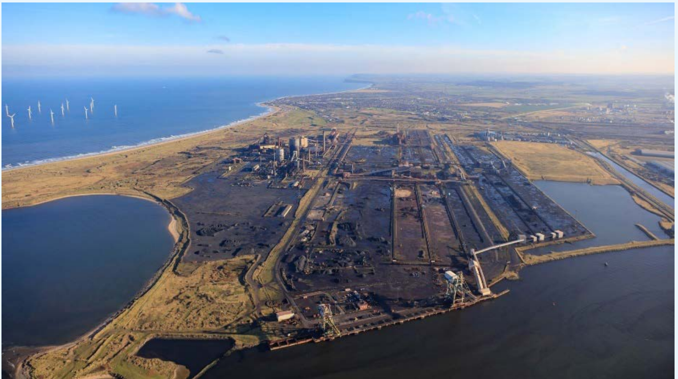
Figure 14: H2Teesside Aerial View
