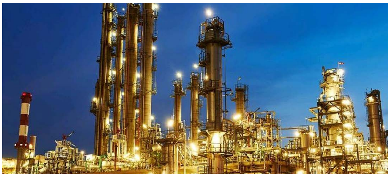
Figure 3: An Autothermal Reforming (ATR) Plant 4
